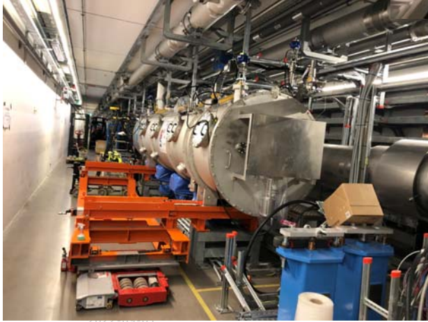
INSTALLATION OF ESS SPOKE, MEDIUM AND HIGH BETA CRYOMODULES -
